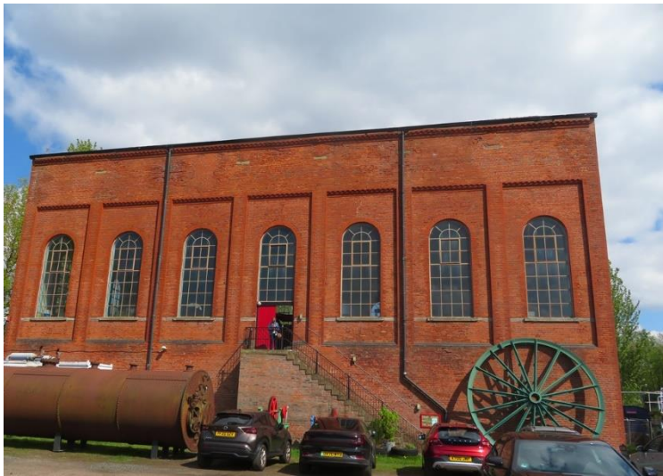
The engine house and (right) showing the the two apertures where the cables connectng to the pit headgear emerged.
