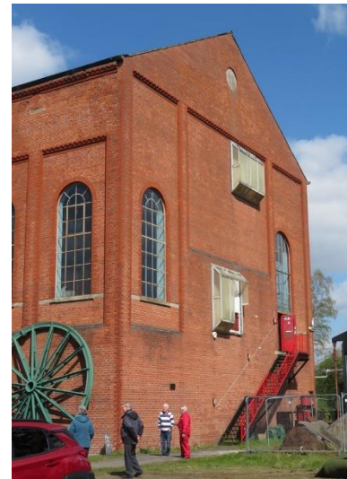
The engine house and (right) showing the the two apertures where the cables connectng to the pit headgear emerged.
